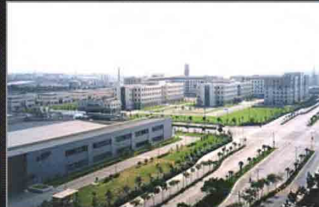
China-Singapore Suzhou Industrial Park, China
