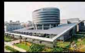
UMCi Wafer Fab Plant
